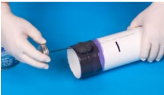
**16.** Immediately, while cement is still wet, assemble the pipe and fittings. If not completely wet, recoat parts before assembly. If cement coatings have hardened, cut pipe, dispose of fitting and start over. Do not assemble partially cured surfaces. While inserting, twist  $1/8$  to  $1/4$  turn until reaching pipe stop. Do not continue to rotate after the pipe has reached the socket bottom.
