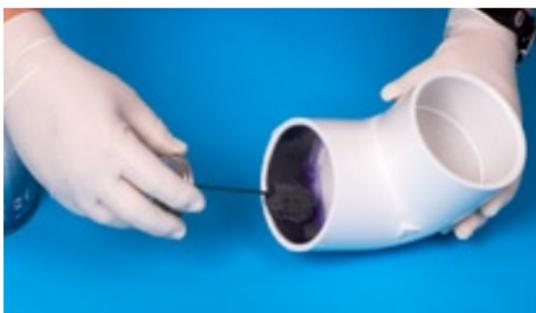
**15.** Apply a second, full even layer of cement on the pipe. Most joint failures are caused by insufficient application of cement.
