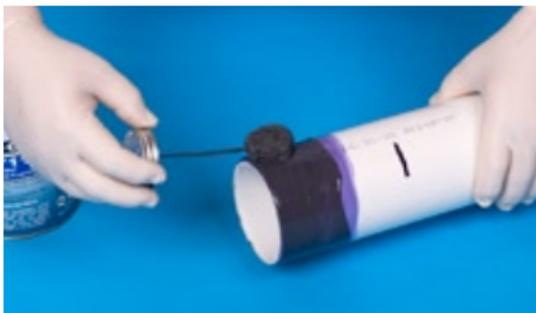
**14.** Aggressively apply a medium layer of cement into the fitting socket; avoid puddling cement in the socket. On bell-end pipe do not coat beyond the socket depth or allow cement to run down into the pipe beyond the bell.
