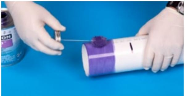
**11.** Apply a second application of primer to the fitting socket. Do not allow primer to run down the inside of the fitting or pipe.
