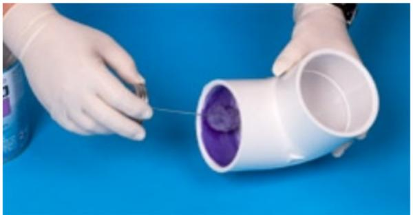
**12.** With the proper size and type of applicator, while surfaces are still wet, immediately apply the appropriate Weld-On cement.
