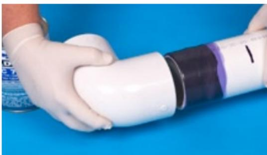
**17.** Hold the pipe and fitting together for a minimum of 30 seconds to eliminate movement or pushout.
